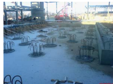
Drilled piers in place
