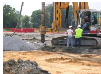
Installation of micro piles
