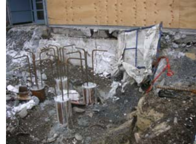
Composite piles in place
