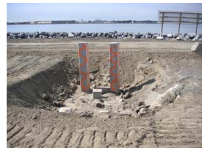
Precast piles in place
