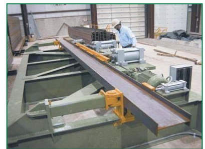
Photo of beam cold cambering.
